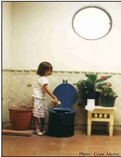
Figure 28 Drying toilet from ESAC/CITA with two vaults. ( http://www.laneta.apc.org/esac/index.htm )
