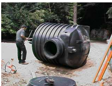
Figure 27 Urine tank in Lambertsühle Material HDP, storage tank ( www.lambertsuehle.de )
