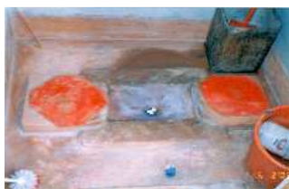
Figure 48 Locally casted urine diverting pan
